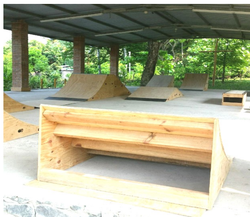
Completed skateboard ramps
