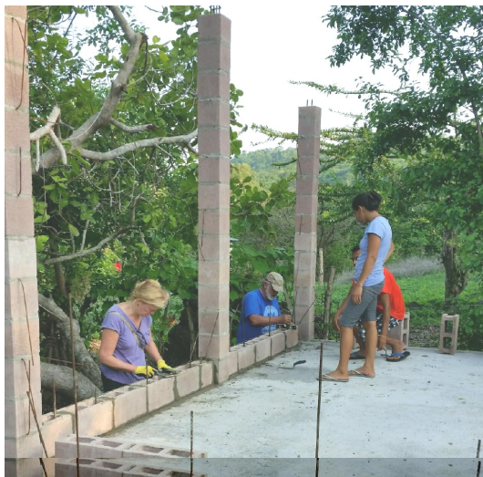
Laying cement blocks for the framework
