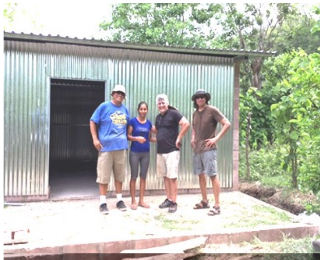
Completed one-room home with tin roof and siding
